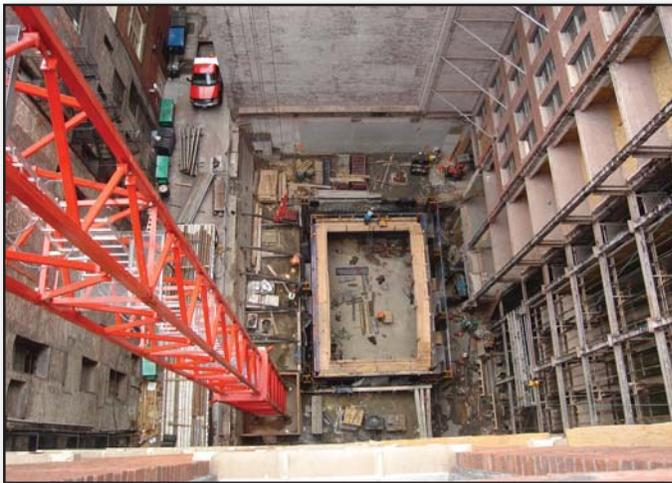
Another unique site challenge was presented during the planning and consideration for placement and design of the tower crane and associated foundation work. Typical concrete pad foundations for a crane large enough to serve the needs of the Alaska Building project carried too large of a footprint for the constraints posed by the building's 104-year-old concrete and granite foundation. Graham successfully designed and engineered (in-house) a 12
